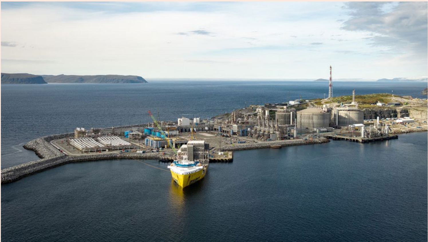
Arrival of the compressor module at Melkøya in August 2026 Photo: Jonny Engelsvoll/©Equinor
