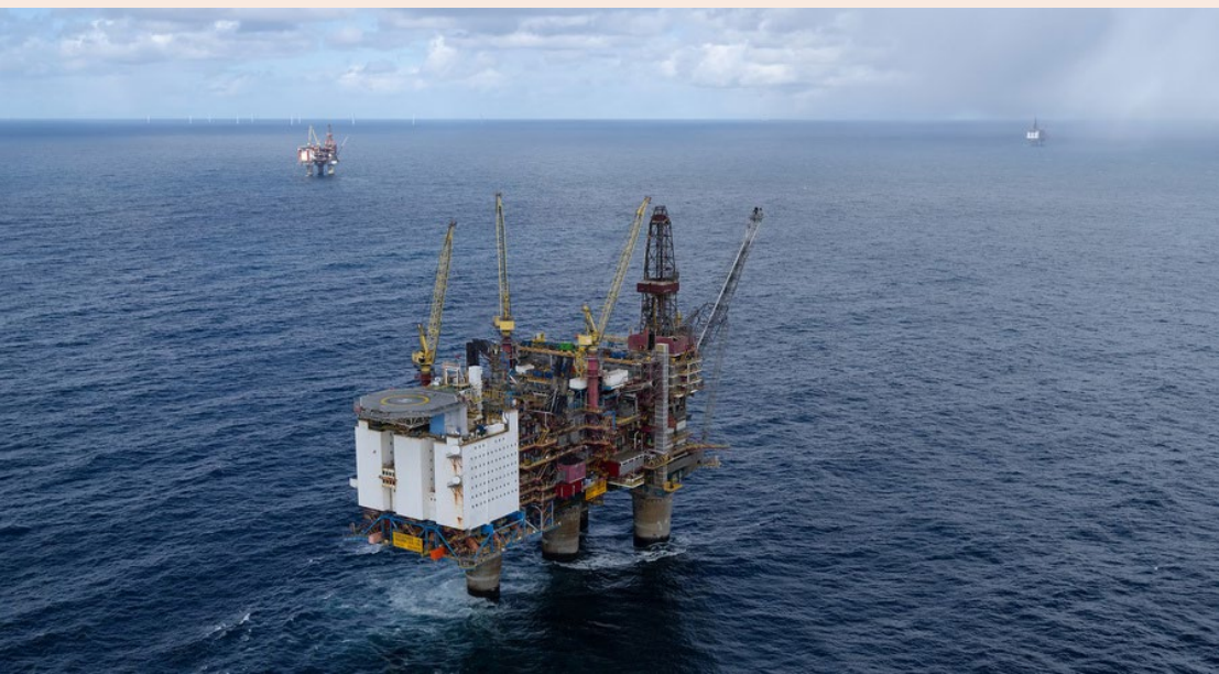
The Gullfaks A platform in the North Sea (Photo: Torstein Lund Eik / ©Equinor)
