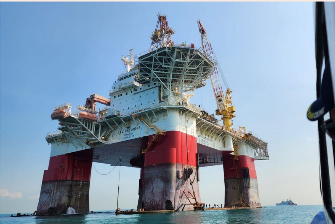
SSV Catarina (Photo source: M3 Marine)
