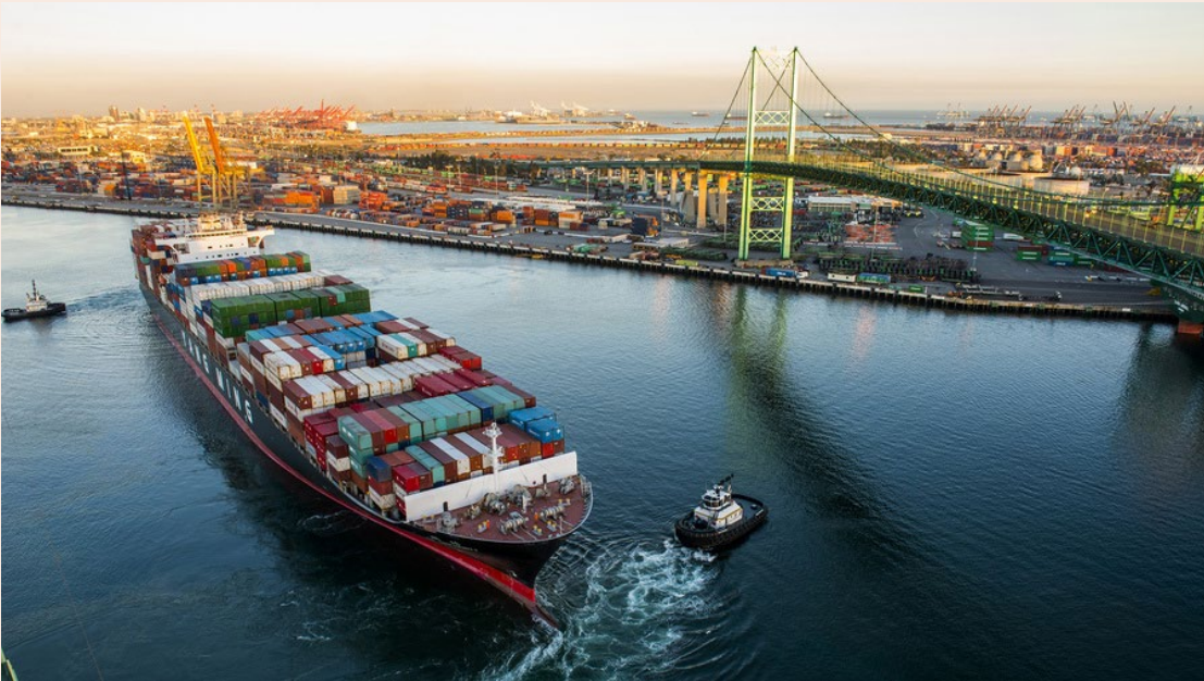
Photo: Port of Los Angeles
