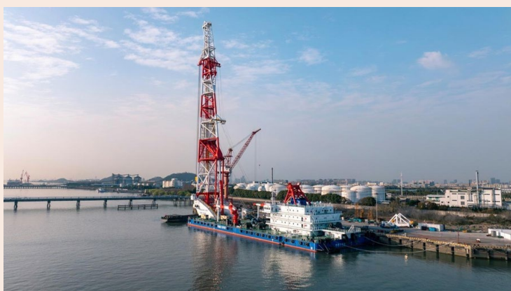
Image Credit: China Railway Construction Bridge Engineering Bureau Group
