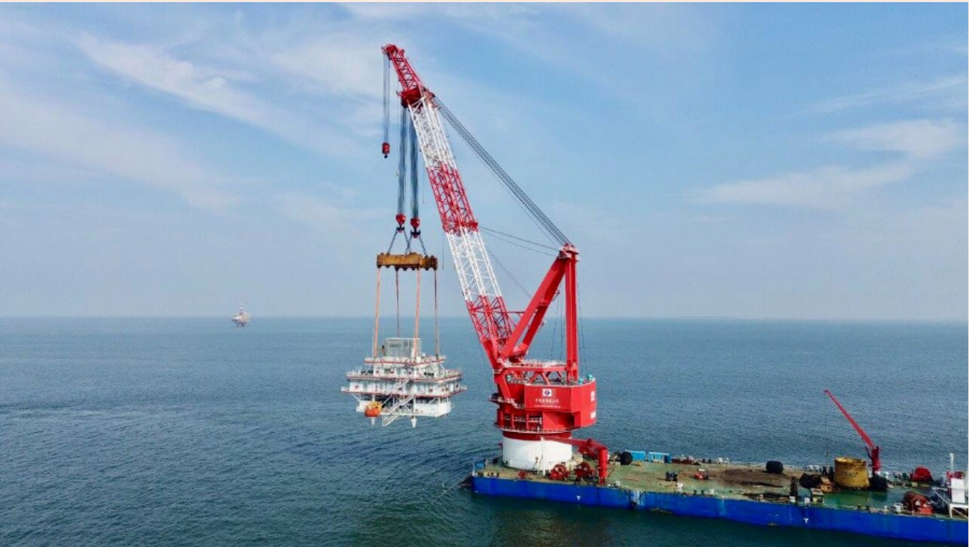
Photo source: Siemens Energy via LinkedIn
