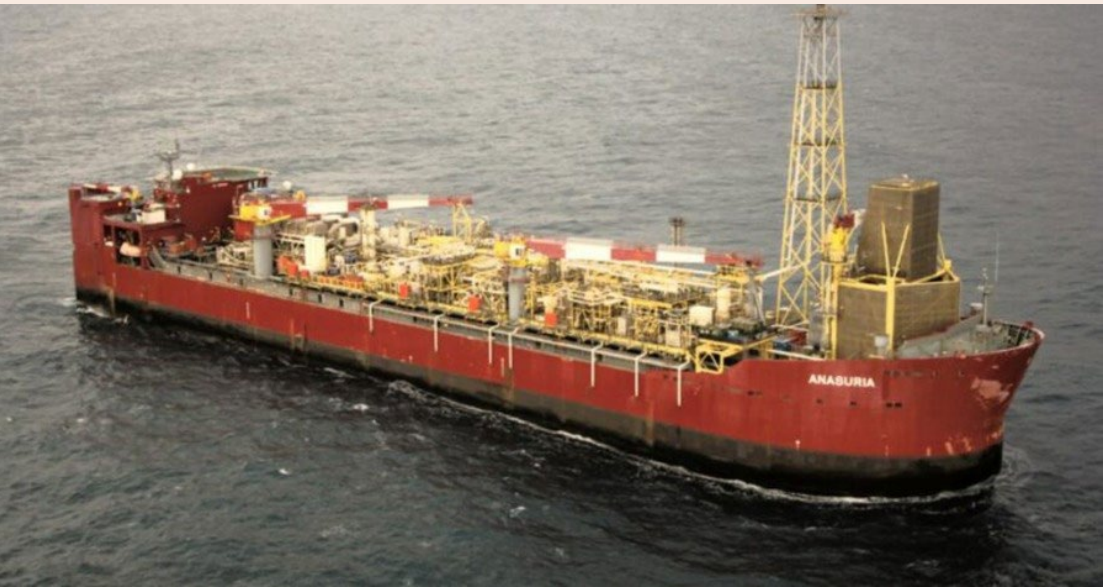
Anasuria FPSO (Photo source: AOC)
