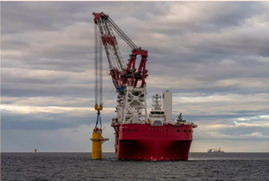
Inch Cape's transition piece installation by Seaway Alfa Lift. (Photo source: Inch Cape)
