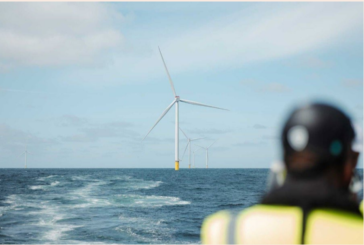
Photo source: RWE
