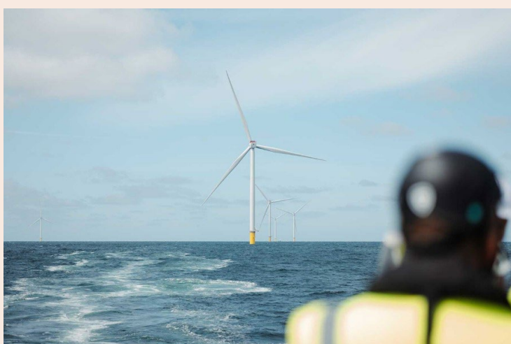
Photo source: RWE
