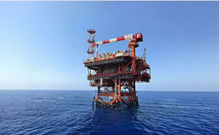
Platform in Zohr field (Photo source: ENI)
