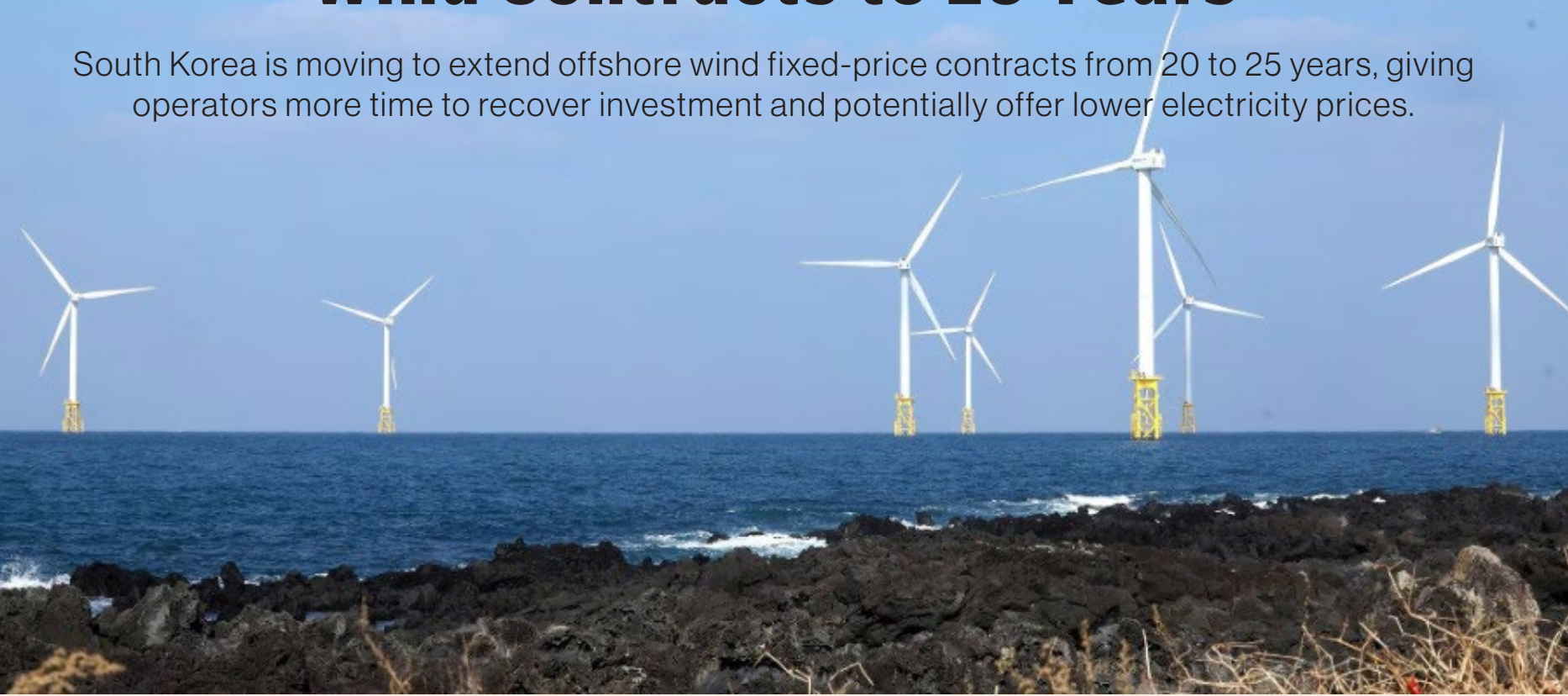
Jeju Hallim Offshore Wind Power (Image credit: Korea Electric Power Corporation)
