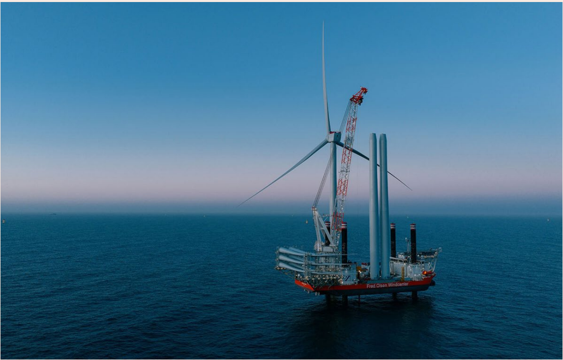
Photo source: RWE
