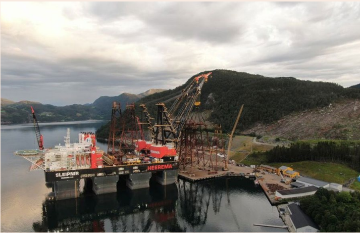
Previous project with Heerema involving module deliveries to AF Environmental Base Vats. (Source: AF Gruppen)
