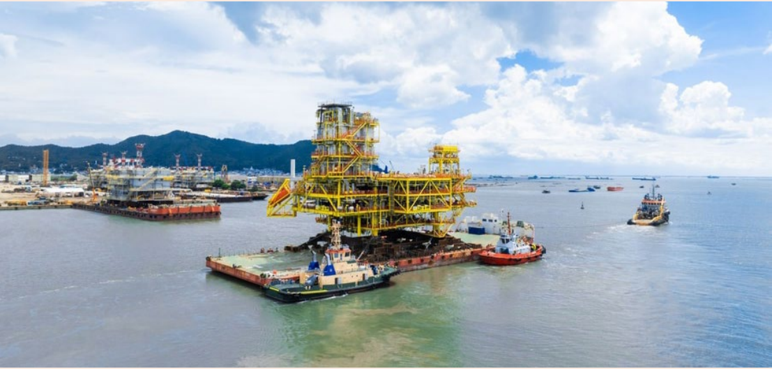
Lac Da Vang platform sail-away (Image source: PTSC M&C)
