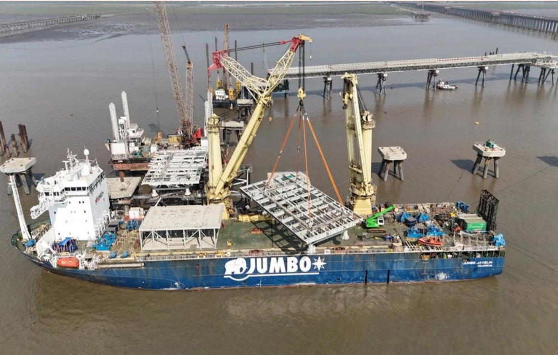
Jumbo Javelin during Dahej berth works. (Image source: Jumbo)
