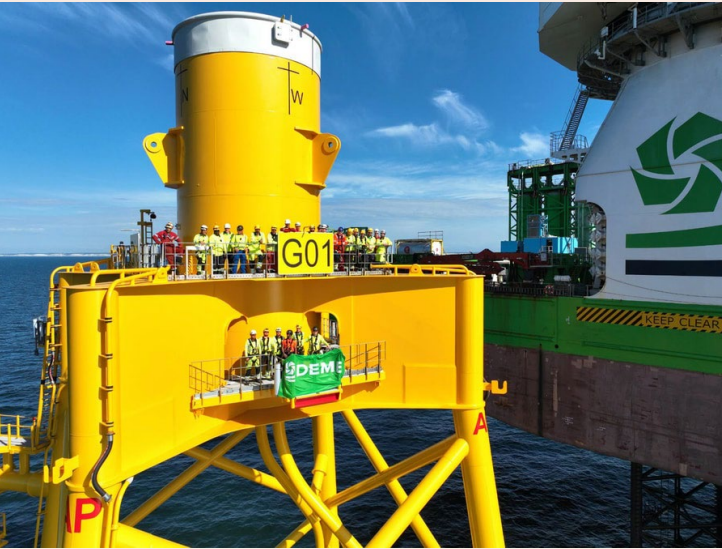
DEME Group completes jacket installation. (Image source: DEME)
