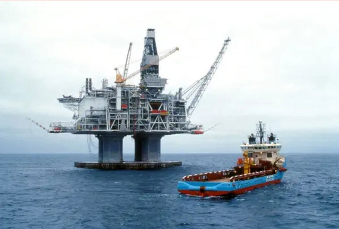
Hibernia Platform (Image credit: Suncor Energy)
