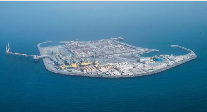
View of the Upper Zakum Artificial Island (Image source: ADNOC)
