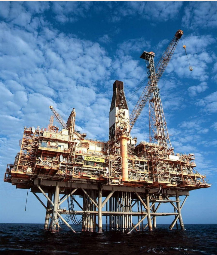
Goodwyn A Platform (Source: Amiga Engineering)
