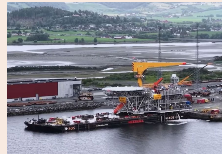
Hugin B topside loaded out at Verdal yard
