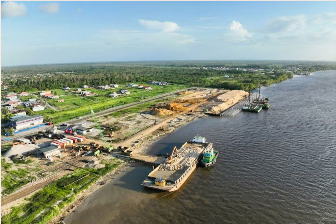
DORDT base supports GranMorgu logistics (Photo source: Saipem)
