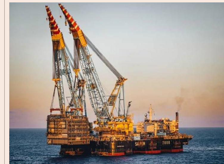
Module installation at Libya's Bouri gas project (Image credit: Saipem)
