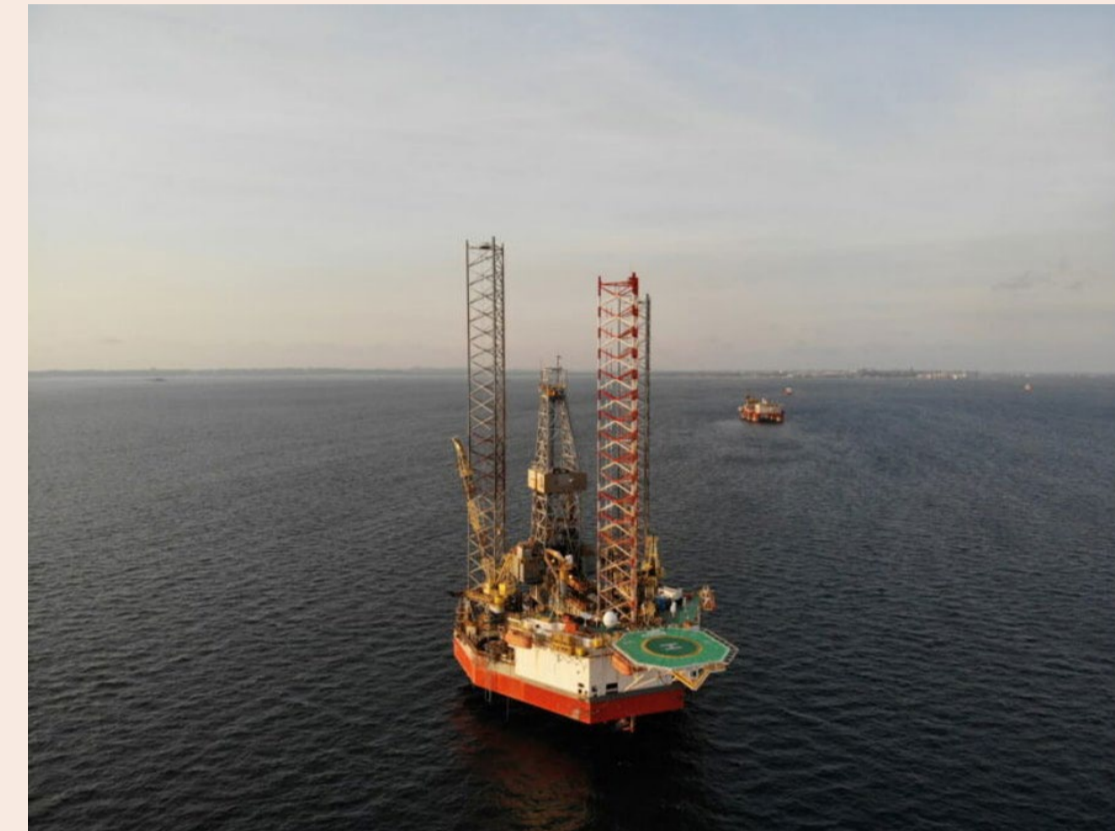
NAGA 6 jack-up rig
