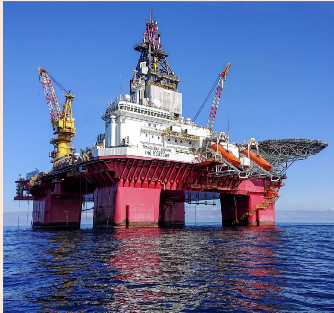
Semisubmersible rig Transocean Equinox. (Photo source: Esqian)
