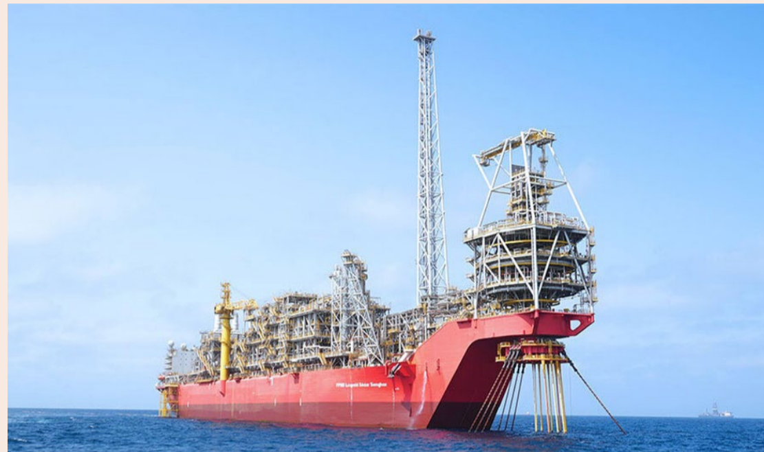
FPSO Léopold Sédar Senghor (Source: Modec)
