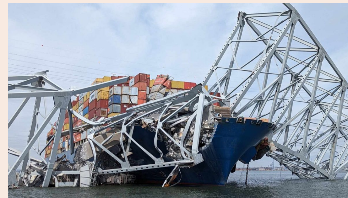
Photo credit: U.S. Army Corps of Engineers, Baltimore District / David Adams
