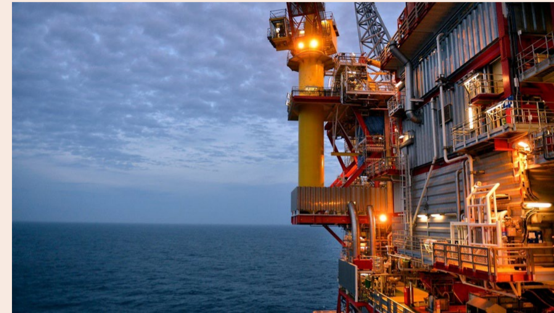
The Kvitebjørn platform in the North Sea. (Photo: Harald Pettersen / Equinor ASA)
