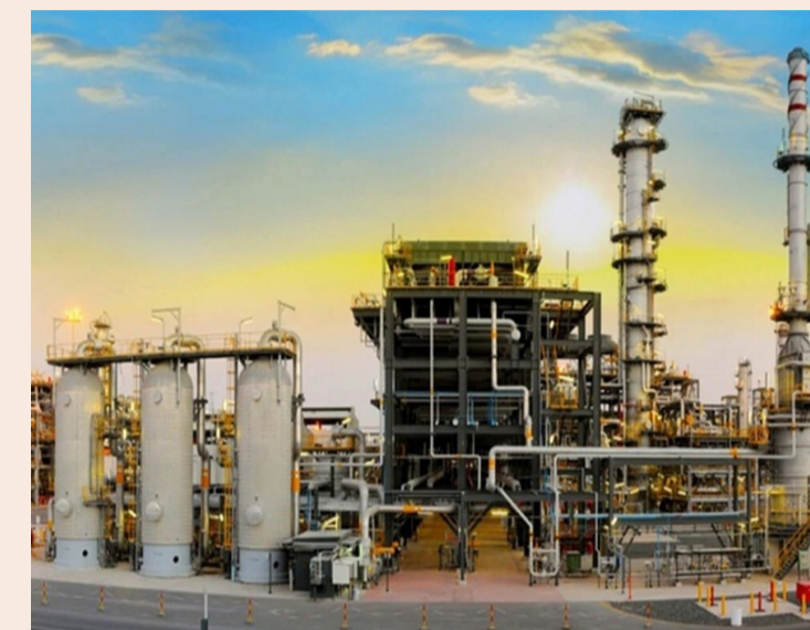
Abu Dhabi National Oil Company (ADNOC) gas processing facility
