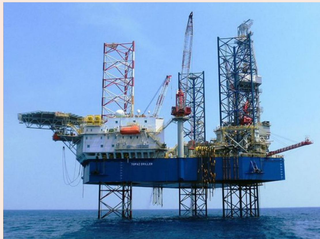
Topaz Driller (Image source: Vantage Drilling)
